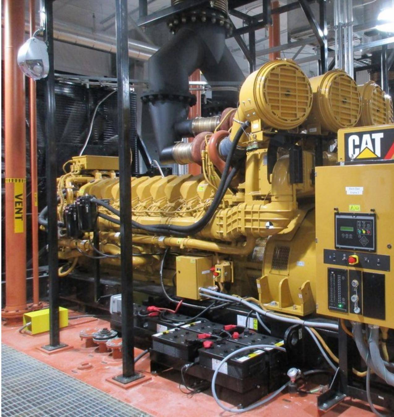
New blackstart diesel engines at the Carroll County Energy Center in Ohio allow the 700-MW power facility to be independently restarted in the event of a widespread grid outage.
